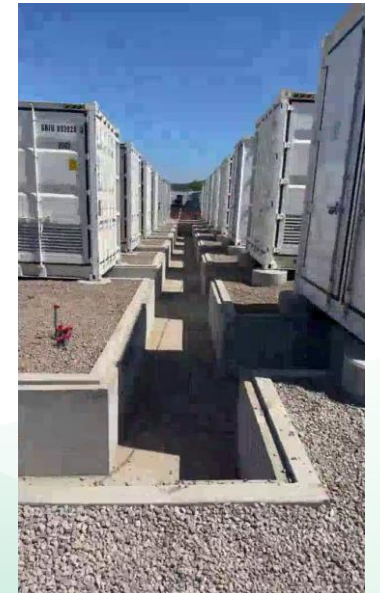
Viejas Microgrid battery yard. Top: Eos batteries. Left: Invinity batteries. Right: Eos trenching.
